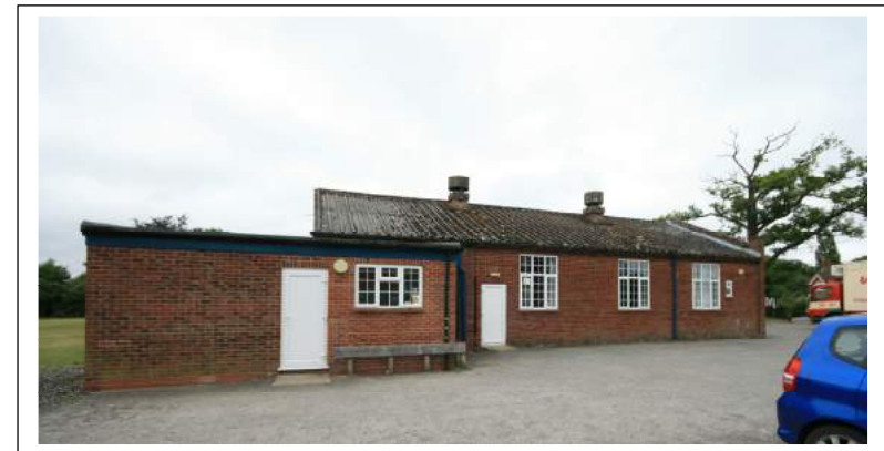
Existing Site - Photographs
